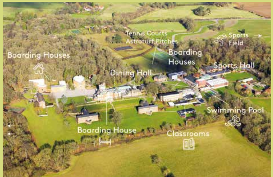
Aerial view of Pangbourne College
