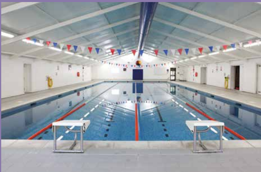
Heated 25 metre swimming pool
